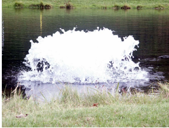
Figure 47: Fountain aeration system; taken from Kasco (2021).
