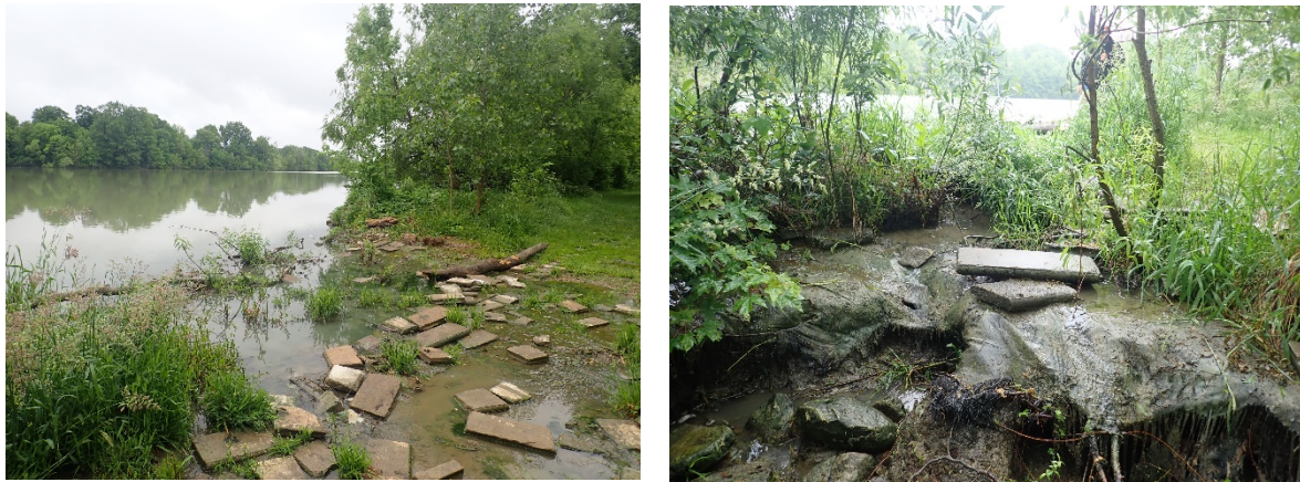
Figure 24: Spillway located along the West Berm looking toward the Lake on top of the West Berm (left) and on the West Ditch side of the berm (right).
