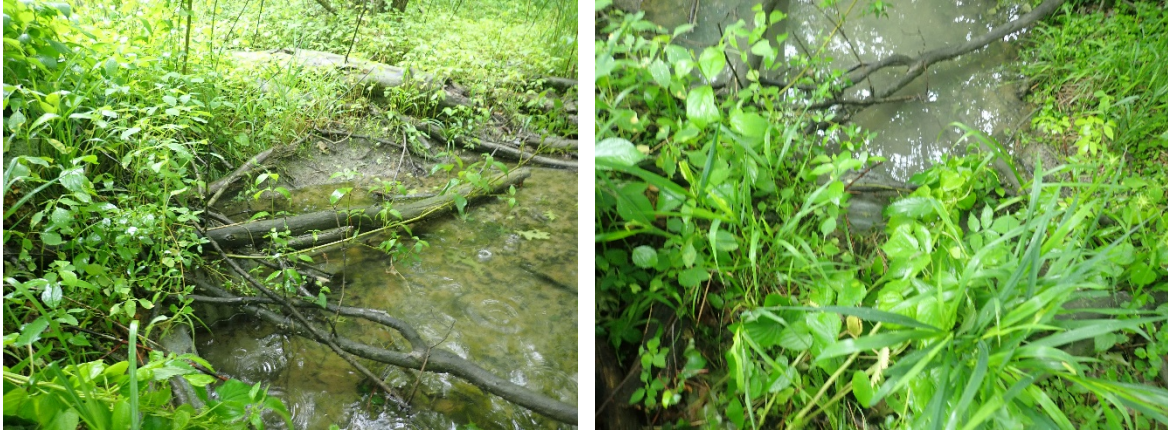
Figure 22: Parallel pipes that convey flow from the Northeast Tributary seen from the side (left) and top (right); location marked as P1 in Figure 20.
