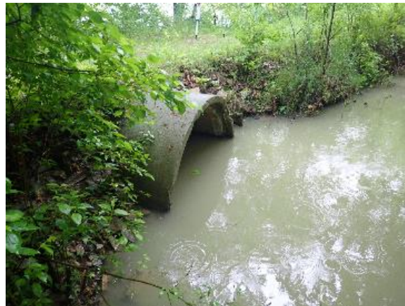
Figure 21: Culvert that is main source of inflow to Olgierd Lake; taken on upstream side of structure; location marked as C1 in Figure 20.
