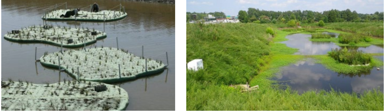
Figure 52: Recently installed floating wetland islands (FWIs) (left) and established FWIs (right); taken from Hunt et al. (2012).
