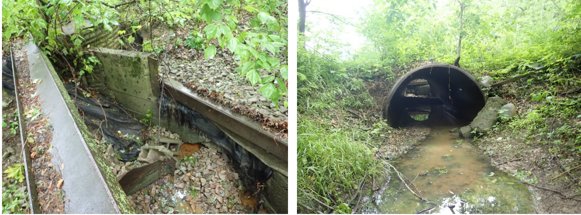
Figure 30: Obstructed weir (left) and culvert (right).
