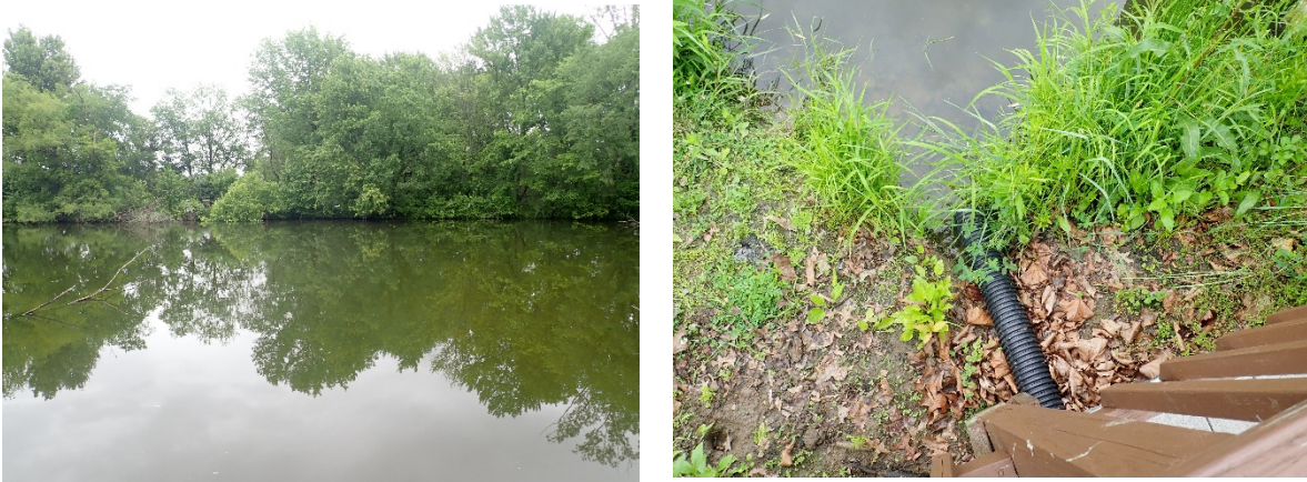
Figure 32: Image of Southwest Pond taken from the dock (left) and corrugated pipe that feeds the Pond runoff (right).
