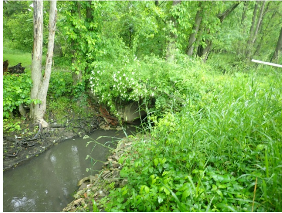
Figure 25: West Ditch culvert (looking upstream); location marked C5 in Figure 20.
