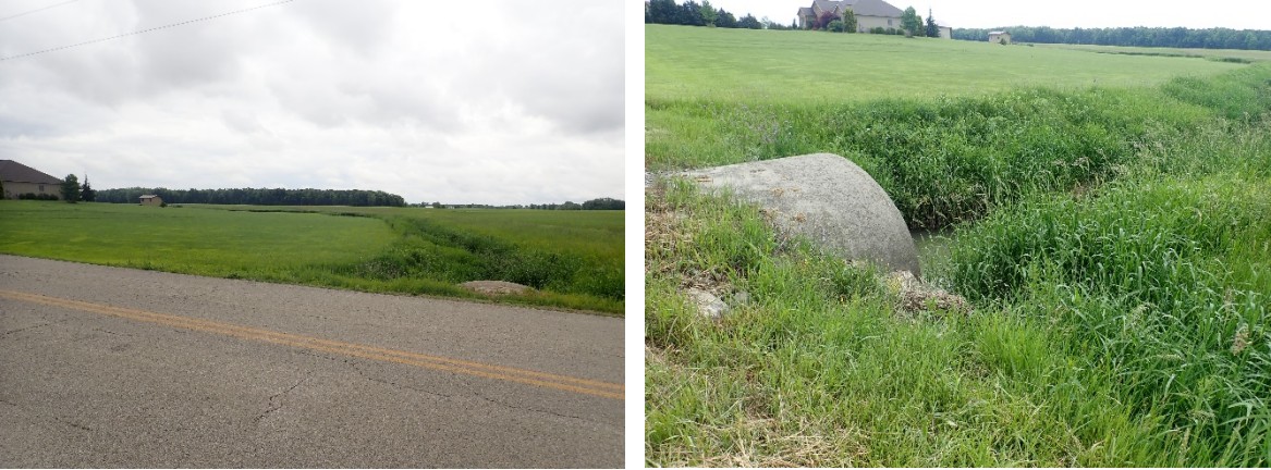
Figure 23: Culvert East County Rd 6 that conveys flow from the Southwest Tributary seen from the top (left) and side (right); location marked as C4 in Figure 20.
